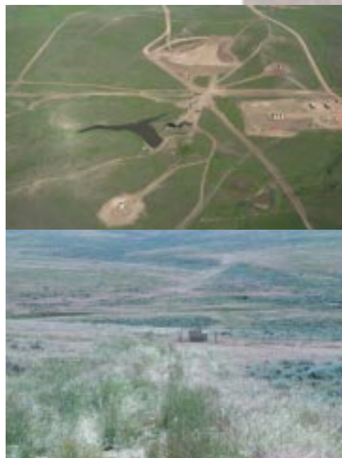
Two views of coal bed methane development.
